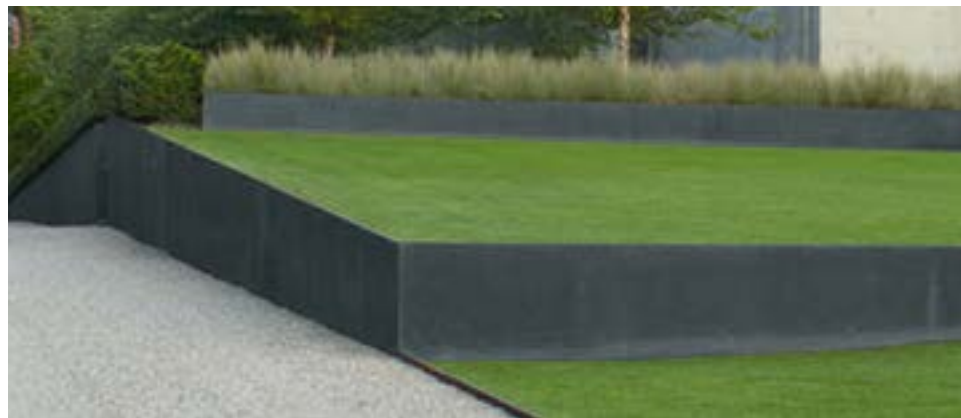
STEEL RETAINING WALLS
