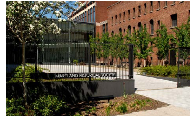
DECORATIVE FENCE AND SLIDING GATES
